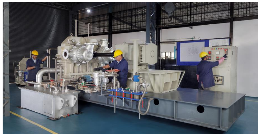
1.8 MW Condensing Turbine under Assembly
